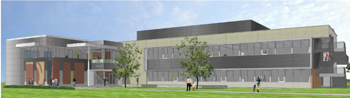
INSTRUCTIONAL BUILDING 1 $18.8 million, new construction Est. Completion: Spring 2021
