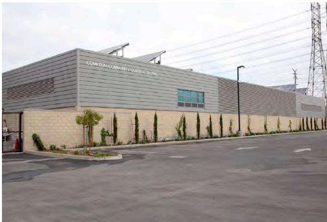
Central Plant and Campus Utility Infrastructure
