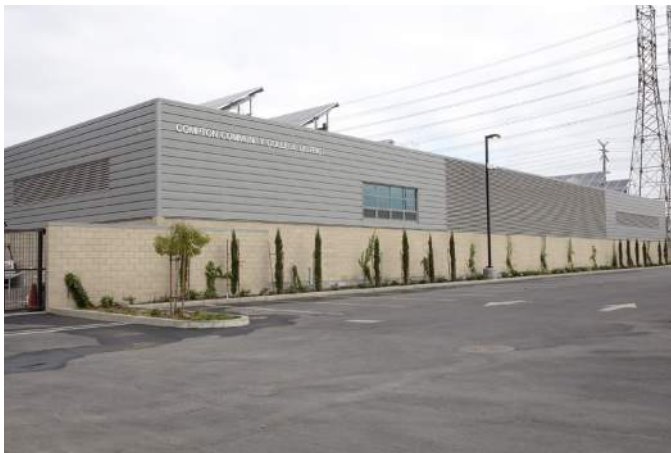
Central Plant and Campus Utility Infrastructure
