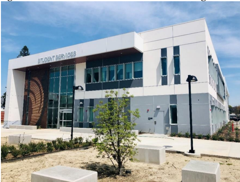
Figure 2: Photo of New Student Services Building
