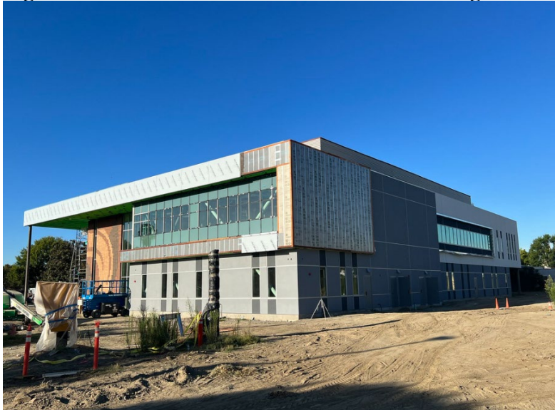
Figure 2: Photo of New Student Services Building Under Construction
